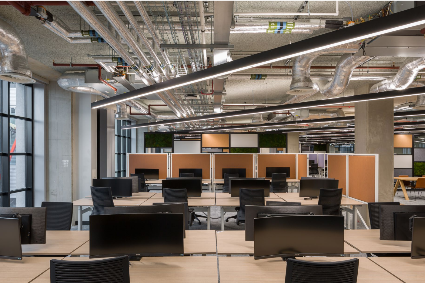
Acospray DC3 in ILA. Manchester Goods Yard
