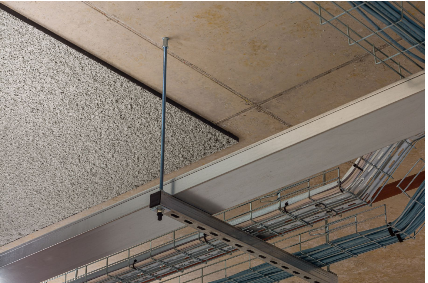
Acospray DC3 in ILA. Manchester Goods Yard
